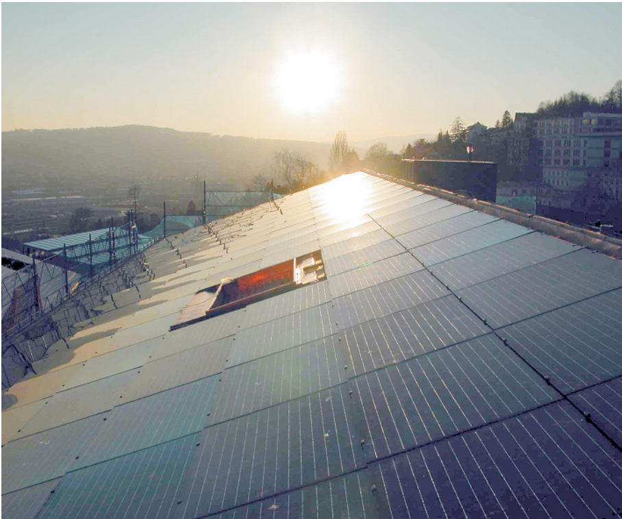
Anlage Application Application Waidspital, Zürich (CH)
